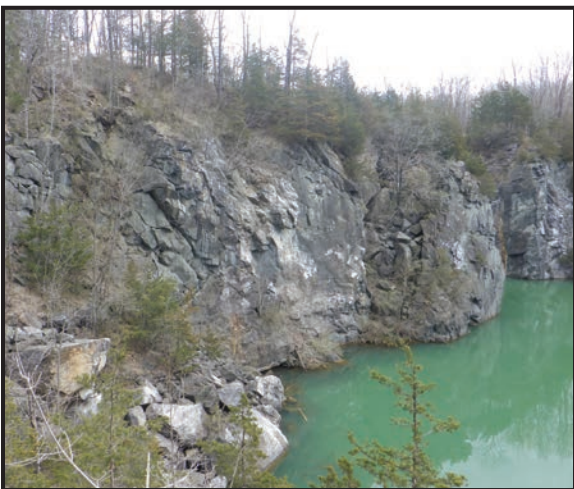
Figure 7. Dike looking east: middle portion is missing, revealing a wall of Franklin Marble. The through-cut into the north chamber of the Taylor Mine is at the far end. Photo by David Vonderheide.
