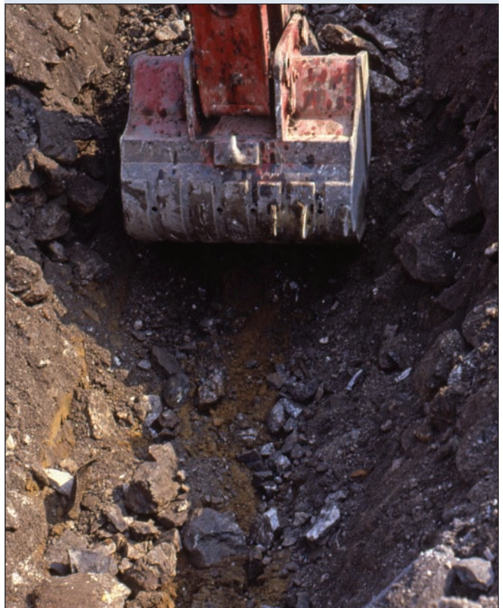
Figure 14. Excavator bucket scouring the bottom of trench as it reaches the ocher-colored clay that gave rise to concern by the New Jersey Zinc Company for the long-term stability of its new railroad trestle.
