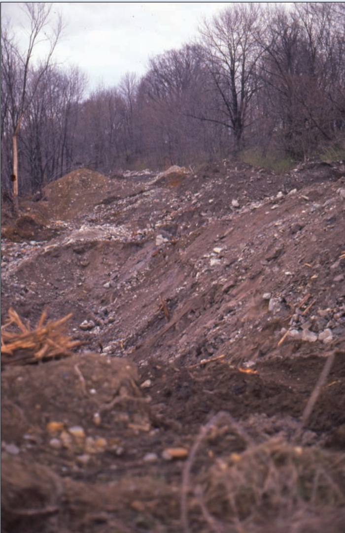
Figure 16. Mine run fill and broken timbers, from the original base of the trestle to the excavated material piled high above, over the length of the site.
