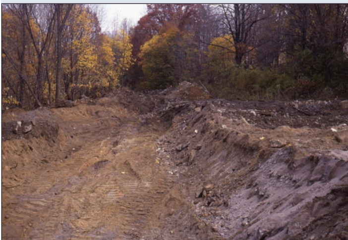
Figure 9. View of exposed mine run fill looking north. Recoverable collecting material diminishes in depth and width as the original ground level rises to meet the old railroad grade.
