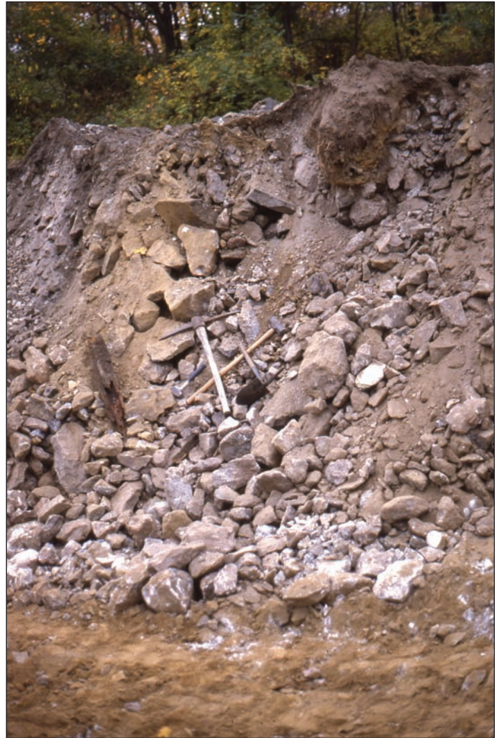
Figure 10. Exposed mine run fill lying between the yet-buried heavy timber supports, seen midway along the former railroad bed. Coarseness, character, and content of the fill varied dramatically, as did its depth.
