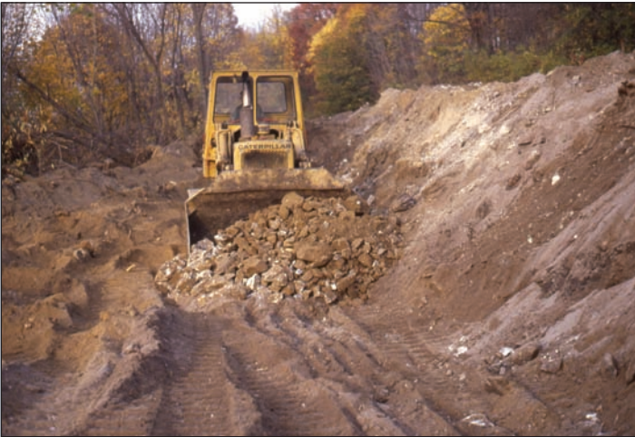
Figure 5. Caterpillar 955 "trackscavator" working at mid-point along the west side of the yet-buried trestle. Mill fines were discarded to the low side. The easily recognizable coarser mine run fill was pushed forward and stockpiled ahead for collecting.
