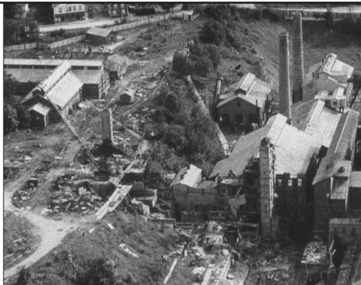
Figure 1. Mill No. 2 being demolished soon after the closing of the Franklin Mine. The storage tanks and crusher building have been taken down. The timber trestle is center left at eight o'clock. Stephen J. (“Itchie”) Novak photo.
