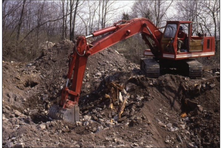
Figure 13. The excavator, working from the original railroad grade, commences excavation of the mine run fill that remains between the still-buried timber trestle supports.
