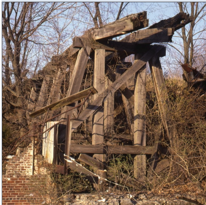
Figure 2. End of timber trestle as it appeared in 1984 at the north side of the Mill No. 2 crusher foundation. Just beyond this point, it was entirely buried beneath mine fill consisting of low-grade ore, gangue minerals, and waste rock.
