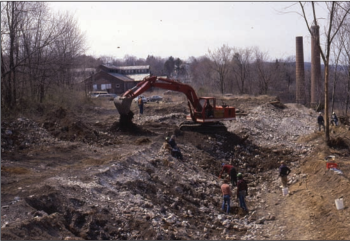
Figure 15. The huge excavator, reaching, digging, scooping, lifting, turning, and dumping its load of mine run fill, as it expands the opportunity for mineral collecting at the Mill Site.
