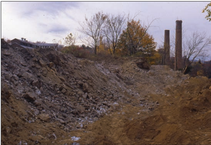
Figure 8. View of exposed mine run fill looking south toward the north end of former Mill No. 2, with powerhouse smokestacks in the background. Timber supports protrude in the distance from stockpiled fill, recovered in its separation from the mill fines.
