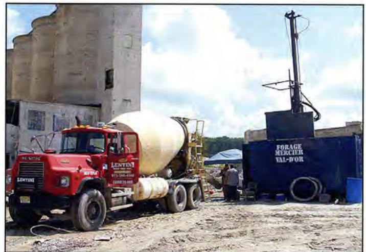
Figure 4. Cement truck grouting and sealing core hole DR2 upon completion of the drilling.
